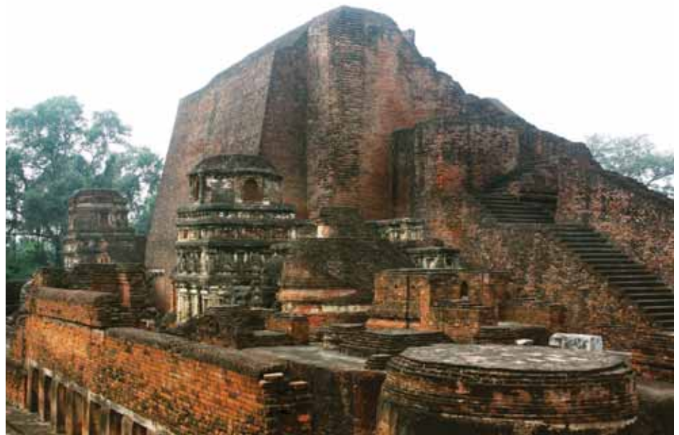
Excavated site of Nalanda, Bihar
